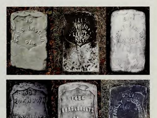
first-generation recessed-shield headstones installed in 1877 and transformed into flat markers in 1934. These photographs illustrate characteristic chipping, cracking, weathering, and staining. The bases were cut or broken off. (Petersburg National Battlefield, 2005.)
