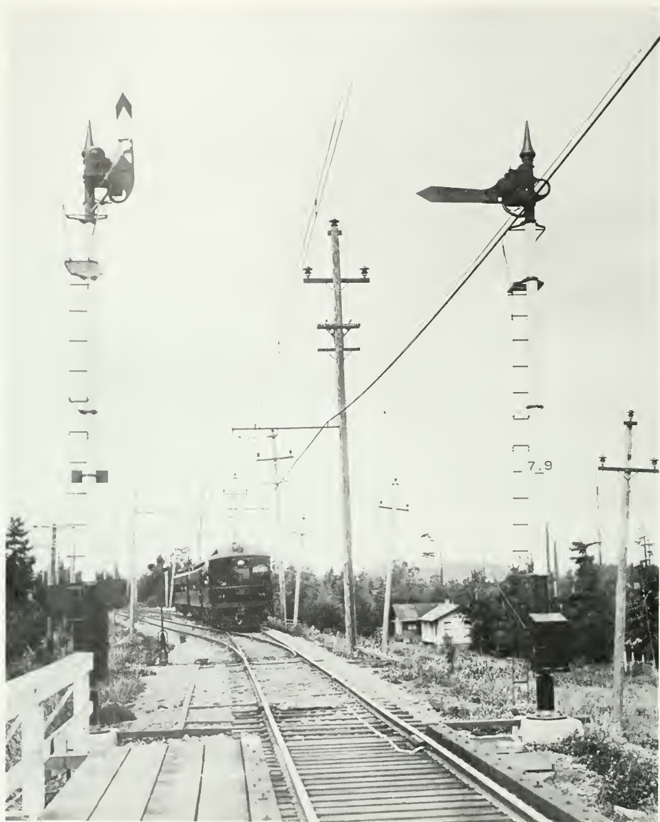
The high construction standards of the Hill-controlled Oregon Electric are evident in this photograph taken shortly after 1910. Heavy rail and crushed rock ballast were employed for trackwork, and catenary construction was used for the overhead trolley wire. On the busiest stretch of OE rail, between Portland and Garden Home, where passenger train movements alone reached a peak of 36 daily, continuous block signals were installed. GENERAL RAILWAY SIGNAL COMPANY.
