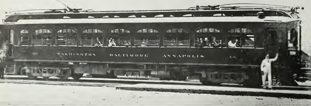
The impressive dimensions of the WB&A's Niles "Electric Pullmans" are evident in a broadside study. The big cars regularly clocked 66-mile-per-hour average speeds once they got out of town. LEROY O. KING COLLECTION.
