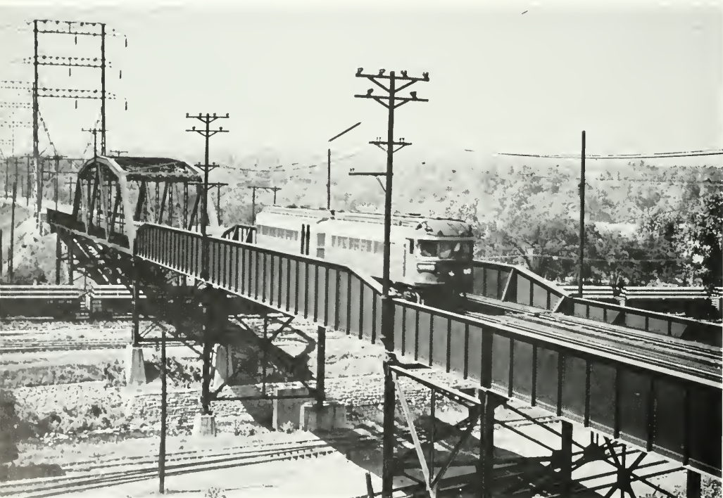
One of the articulated "duplex" units rebuilt by TMR&L shops from conventional equipment in 1929 crossed the substantial steel structure that carried the rapid-transit route over the Menomonee River and the Milwaukee Road main line. WILLIAM D. MIDDLETON.
