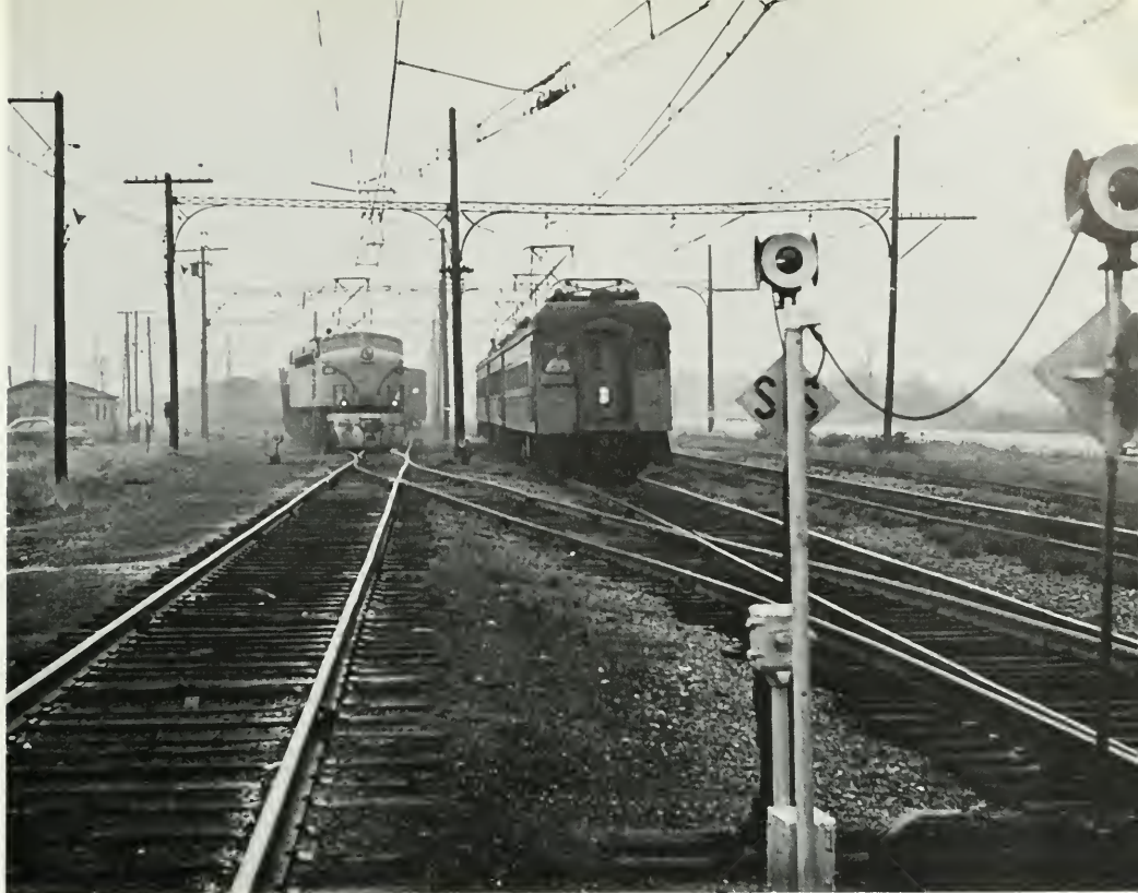
Eastbound with afternoon commuters in 1955, a Michigan City train pounded past Burnham Yard near Hammond, Ind., where one of the South Shore's three 273-ton "Little Joe" locomotives made up an eastbound freight. WILLIAM D. MIDDLETON.
