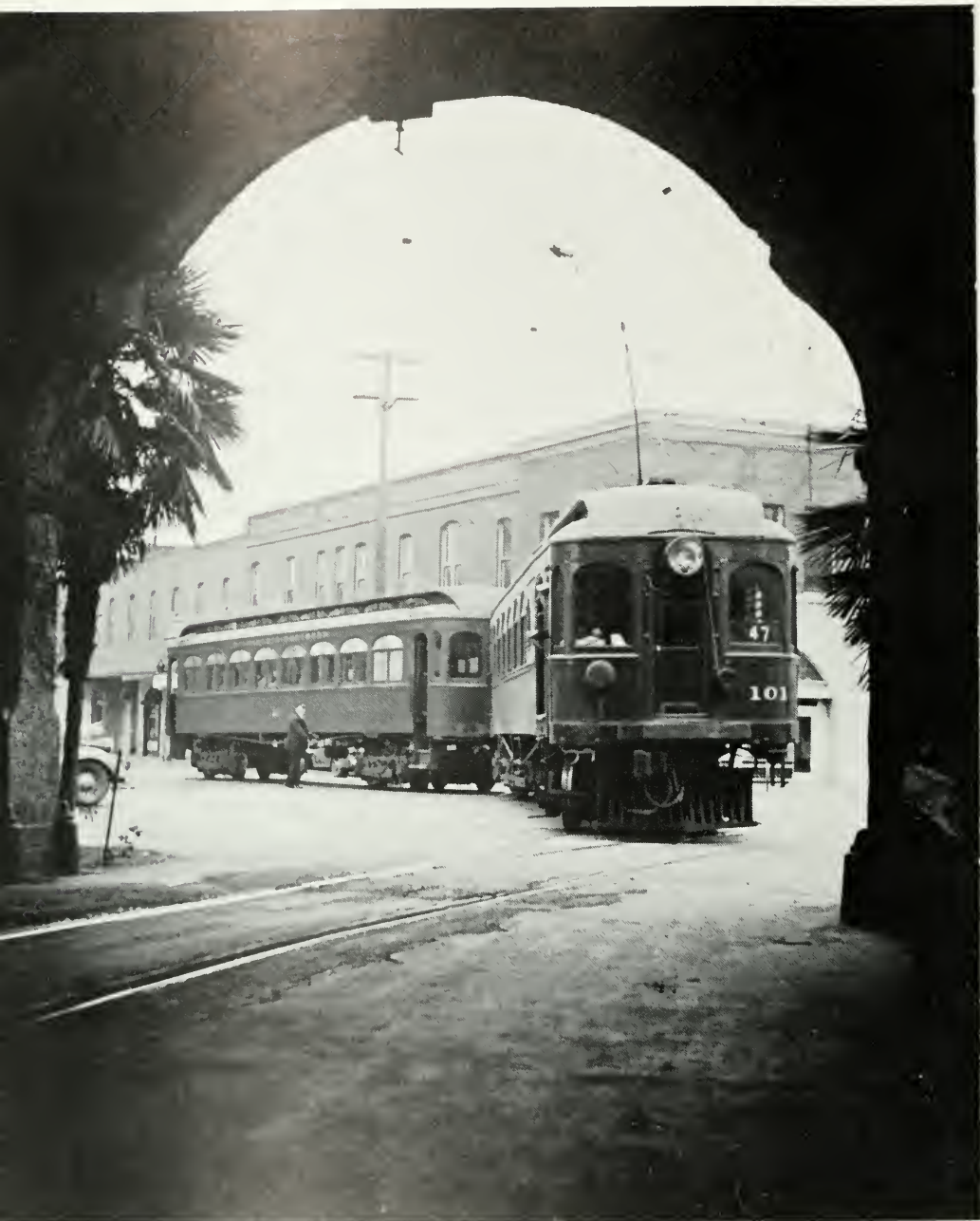
One leg of the SN turning wye in Woodland was under the station arches. Train 47 was heading for a connection with the westbound Comet. B. H. WARD.
