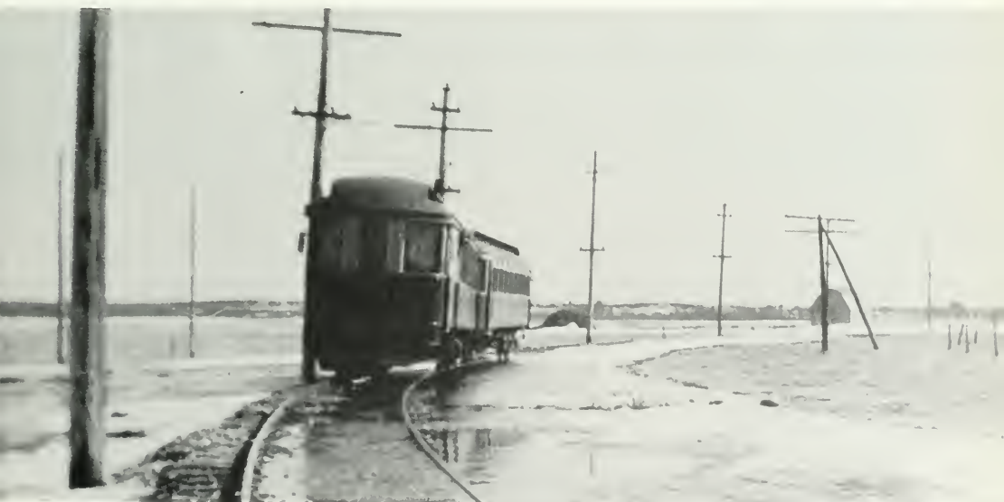
In April of 1929, the winter's snow melted and produced a severe spring flood, causing this two-car train on the Stonewall line to make its way cautiously through water that lapped at the rails. STAN F. STYLES.
