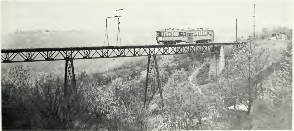
A bright orange West Penn interurban rambled across the high bridge at Brownsville. The broad-gauge system lasted until the mid-'50's, despite a lack of commuters and carload freight. DAVID A. STRASSMAN.
