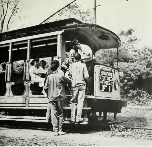
Excursionists boarded a restored Connecticut Company open car in 1959 for a ride over the Branford museum's line near East Haven, Conn. WILLIAM D. MIDDLETON.
