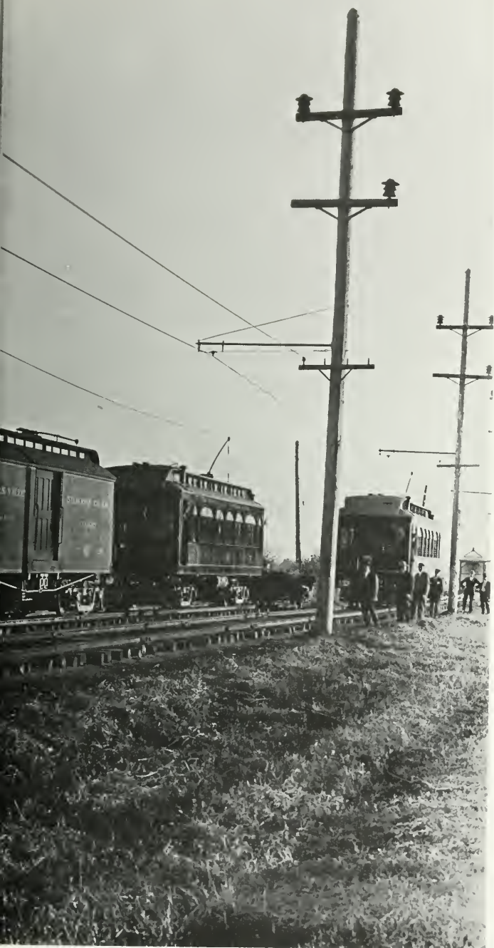
A line-up of equipment was photographed just outside Hutchinson, Kans., on the opening day of through service to Wichita by the Arkansas Valley Interurban Railway in 1915. The complete absence of ballast was a condition that, unfortunately, remained permanent on much of the AVI. Car No. 6, in the foreground, expired in spectacular fashion in 1928 when it was wrecked and burned in a high-speed head-on collision with a freight train. WILLIAM J. CLOUSER COLLECTION.
