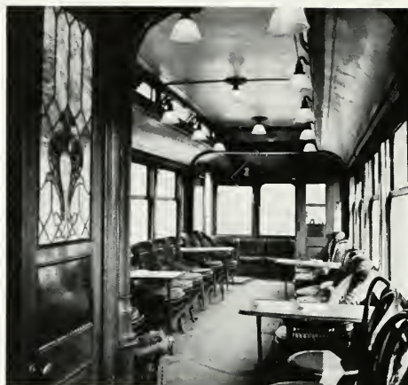
Connecticut Company officers and other distinguished personages rode about the system in high style aboard business car No. 500, built in 1904 by the J. G. Brill Company. The car's interior was finished in hand-carved oak, provided with a lavatory and steward's galley, and furnished with broadloom carpeting and wicker lounge chairs. After the end of Connecticut Company electric passenger service, No. 500 became the première car of the Branford Electric Railway museum, where these photographs were taken in 1959. BOTH PHOTOS: WILLIAM D. MIDDLETON.
