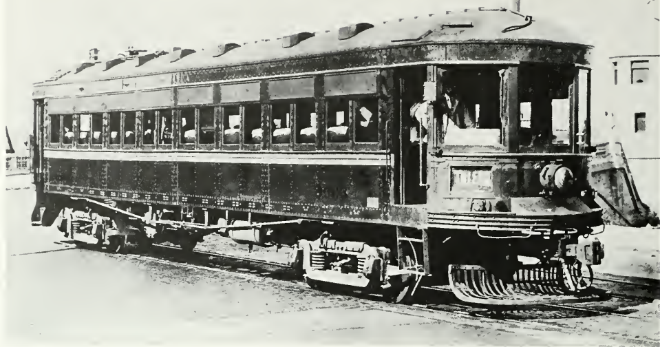
The company's glittering parlor car 7500, available for official duties or charter service, was fitted with deep solarium windows at the front end and this elegant observation platform at the rear. GEORGE KRAMBLES COLLECTION.
