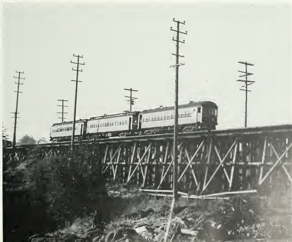
Highlighted by the morning sun, three cars full of BCER commuters hurried across Gladstone Trestle on a 12-mile run from New Westminster to Vancouver over the Central Park line. STAN F. STYLES.
