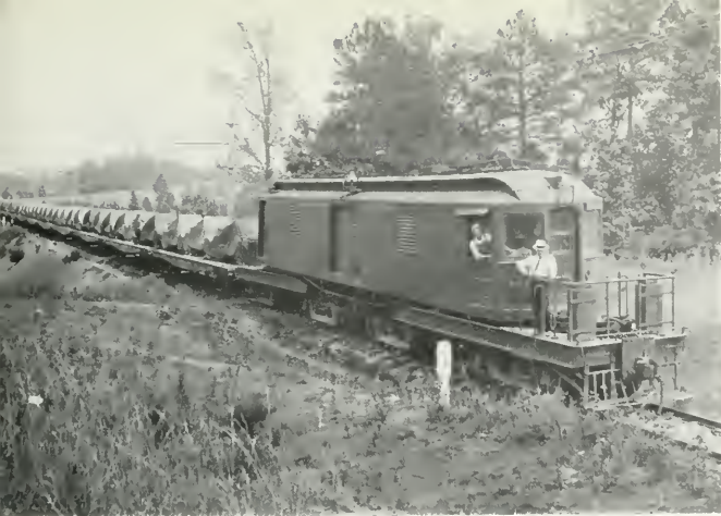
Wooden-bodied 5502, built in the Piedmont & Northern Railway's Greenville (S. C.) shops, hauled new Buicks around 1916. This was one of the first interurban locomotives of the four-truck, articulated-frame pattern. PIEDMONT & NORTHERN RAILWAY.
