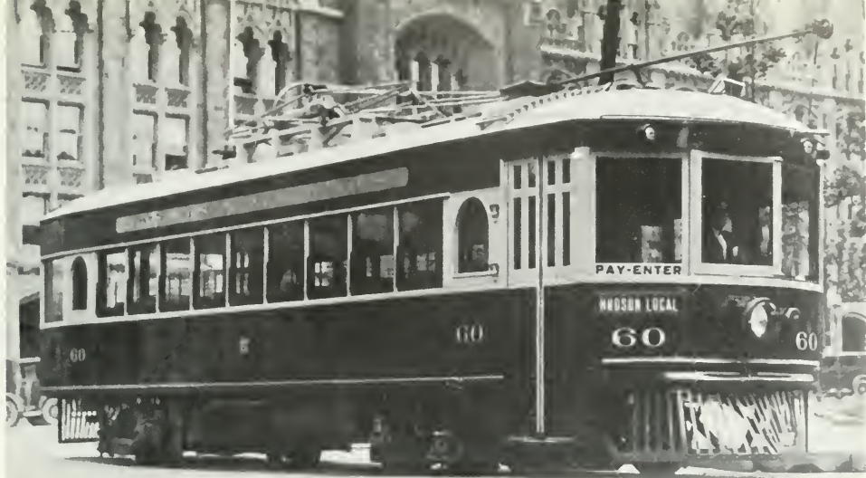
Albany-Hudson Fast Line No. 60 was well equipped for current collection, with trolley poles, pantograph, and third-rail shoes. The Fast Line was abandoned in 1929, but this car rolled up the miles until after World War II, on the FJ&G and on the Portland-Oregon City interurban. JOHN D. MURPHY, FROM WILLIAM R. GORDON.
