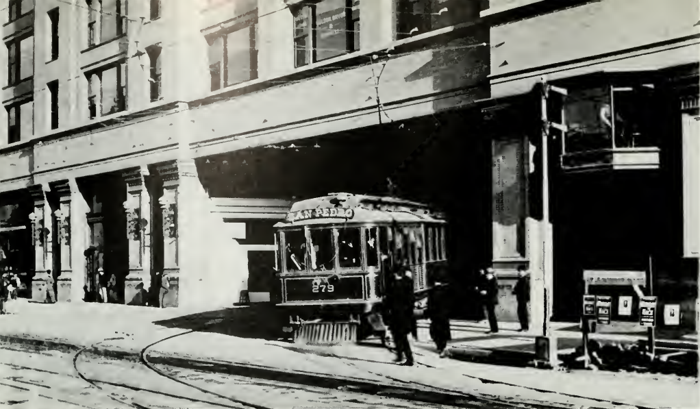
Both the Sixth and Main Street terminal building and the San Pedro interurban line were new when this photograph was taken about 1906. No. 279, scraping the pavement as it beeled into the terminal, was one of 130 semi-open cars delivered by the St. Louis Car Company between 1902 and 1906. The sidewalk semaphores and track switches were operated from the raised bay-window office to expedite heavy two-way movements in this then stub terminal, and to protect narrow-gauge city cars which also used Main Street's three-rail trackage. AL HAJI COLLECTION.
