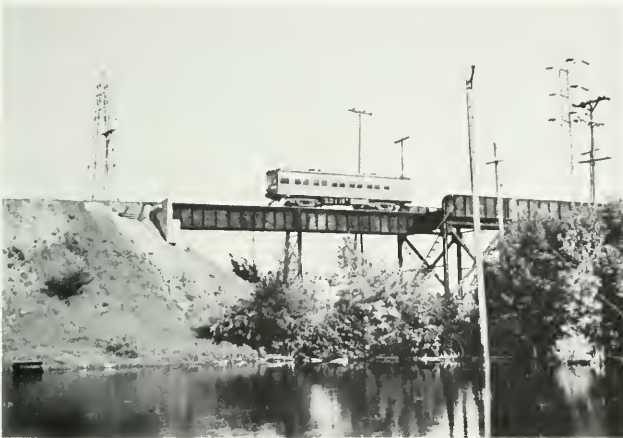
Inbound from Hales Corners in 1949, a Milwaukee Electric interurban crossed over the Chicago & North Western at West Junction on a bridge that was clearly constructed to accommodate future multiple track. The structure was part of a mile-long cutoff completed in 1927 which afforded Burlington and East Troy interurbans access to the new rapid-transit entry to Milwaukee, cutting 23 minutes from previous running times via city streets. WILLIAM D. MIDDLETON.
