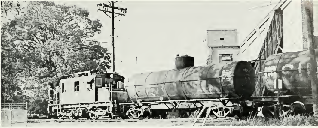
To augment the motive power available for its growing freight traffic, the Sand Springs purchased two 43-ton locomotives from the Niagara Junction Railway of New York in 1946. One of the radio-equipped steeple-cabs, No. 1006, pulled a cut of tankers from the Sinclair plant at Sand Springs in 1954. WILLIAM D. MIDDLETON.
