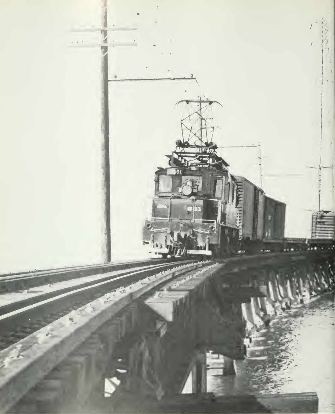
The flatland running that carried Sacramento Northern trains from the Suisun Bay ferry to Sacramento was broken by the 2-mile Lisbon trestle which crossed the Yolo Basin. Such was the quality
