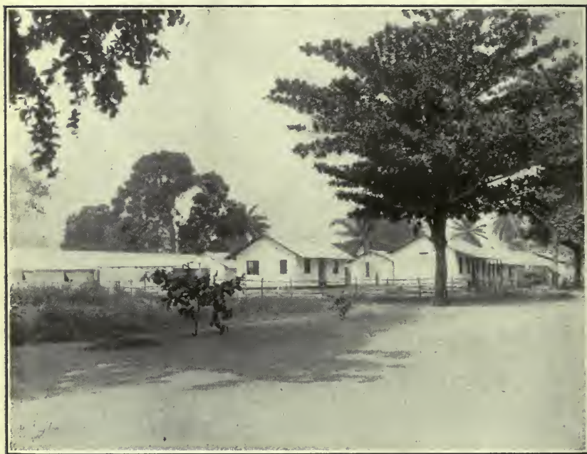
HUTTED HOSPITAL, DUALA.
